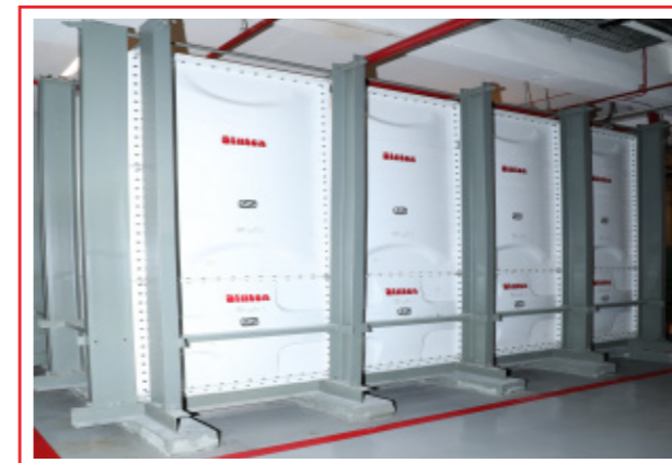
48,000 litres SMC Panel Tank - Moxy Hotel, Bengaluru
